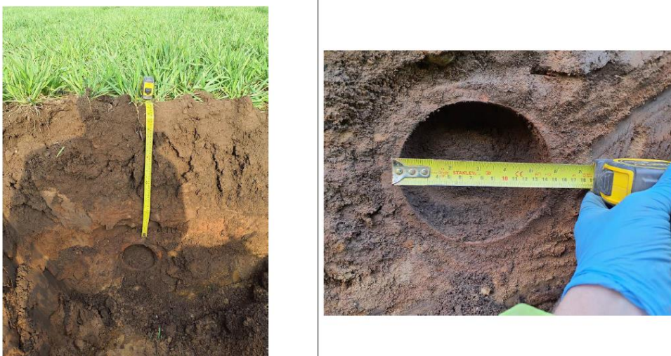
Figure 2: Existing Buried Pipe
