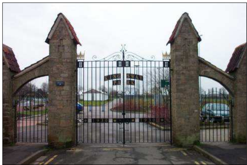
Main entrance gates off Hodgkinson Road
