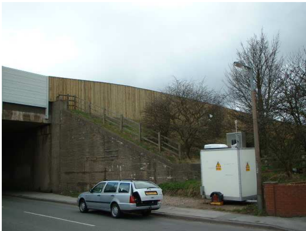
Noise Attenuation Barrier erected across the bridge over the M1 Motorway at Pinxton Green
