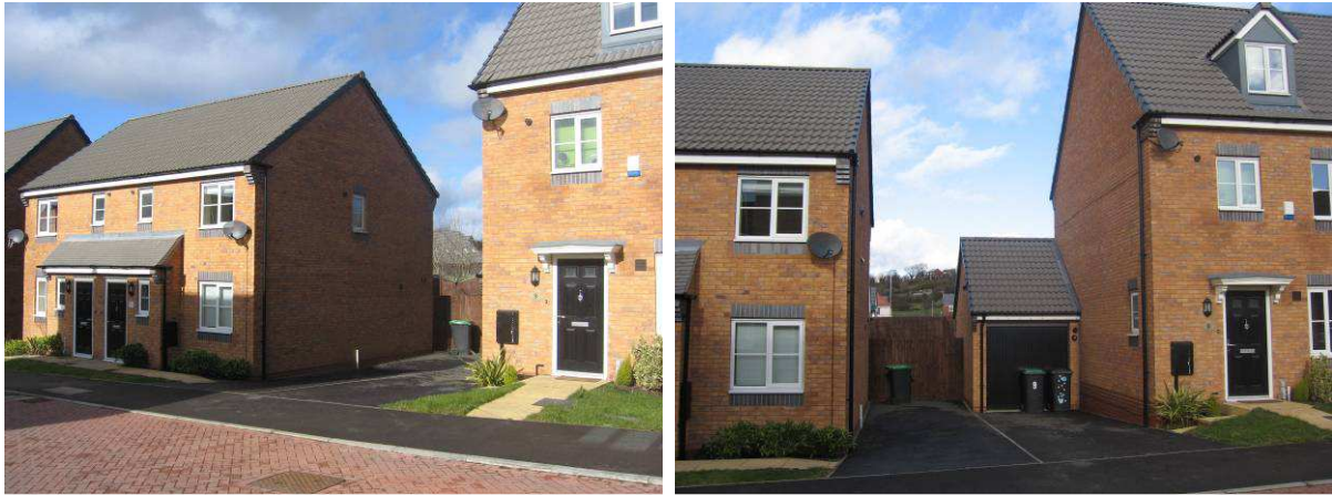
Parking discretely positioned between houses minimising the visual impact on the street scene
