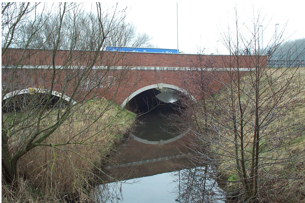
Figure 3: River Maun inlet culverts at the upstream end of Kingsmill Reservoir
