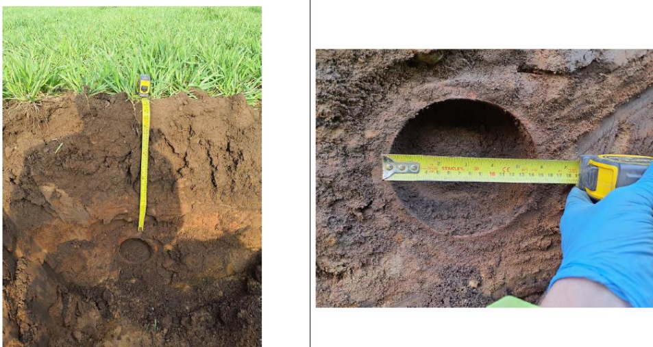
Figure 2: Existing Buried Pipe
