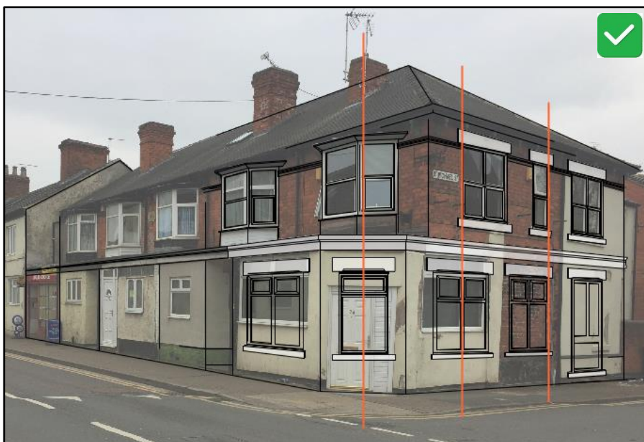
Preferred arrangement. Lower floor windows are aligned with the upper floor and window heads are replicated.
