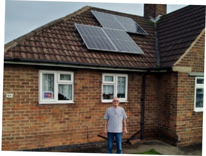
Huthwaite tenant benefiting from new solar panels
