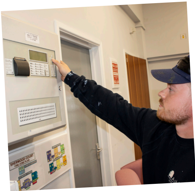
Housing repair technician inspecting a fire board
