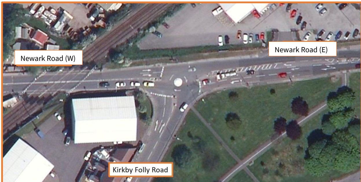
Figure 17: existing Newark Road/Kirkby Folly Road mini-roundabout
