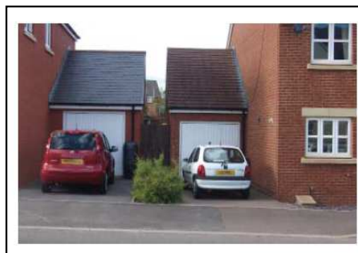
Example of good design with drives/garages located to the side, minimising their visual impact.
