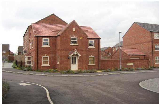
Building turns the corner with active frontages to both streets
