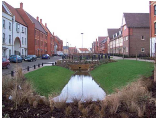
Manual for Streets identifies that SuDS systems Can be successfully incorporated into streets (Andrew Cameron, WSP)
