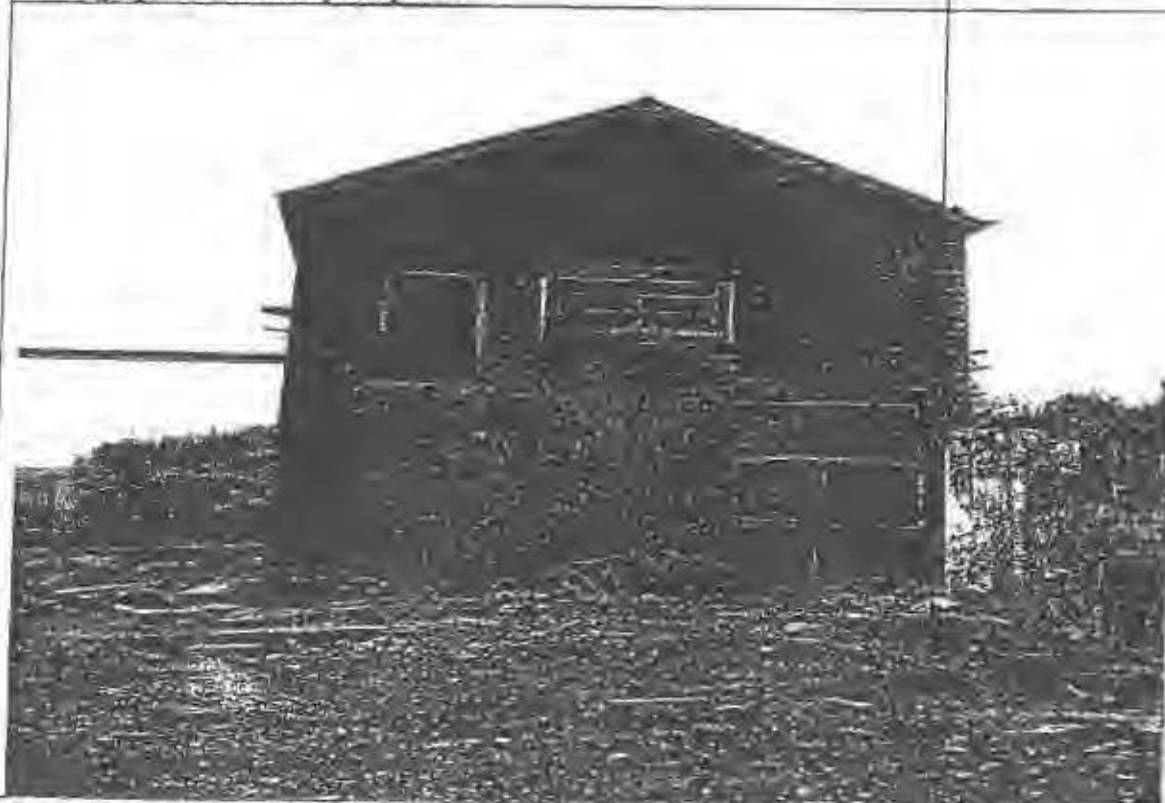
Photograph 2: Electricity Shop North
