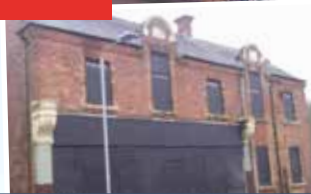
Middlebrook Road, Underwood before redevelopment
